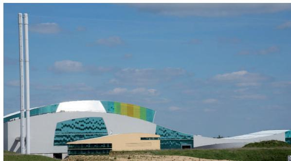
Opened in 2013, Ardley EfW processes around 300,000 tonnes of non-hazardous, post-recycling and residual waste. One of the challenges included a 12m deep basement built over an Artesian Well, alongside requirements for waterproofing, grouting, flooring and sealant work. Working with Tata Projects, Fosroc ensured the specification for the scheme was robust and crucially buildable.
