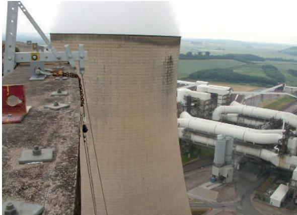
External refurbishment was required to five of the eight steel-reinforced concrete cooling towers. The towers are 118m tall, with a base diameter of 95m, 45m at the top and 37m at the neck. The 40-year-old structures required a repair mortar that could protect from further carbonation and could be applied in thicknesses in excess of 50mm. The material needed to be lightweight due to the difficult application conditions.
