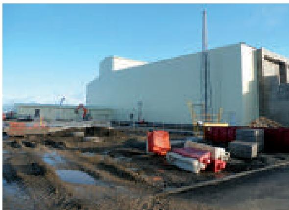
The construction of a convertor station on Deeside was required as part of the £560m interconnector project, designed to link the Irish and UK electricity grids. The contractor faced issues of ground subsidence, gas contamination and water ingress associated with high tides. Fosroc provided a solution encompassing water and gas proofing, joint sealing and concrete repair.
