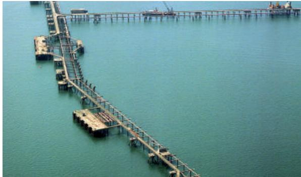
At South Hook, as part of the repair and strengthening of existing jetty and mooring structures, a cathodic protection system was installed. A compatible, sulphate resistant, cementitious material was required to cover a surface area of 14,000m<sup>2</sup>, at a thickness of 25mm. Fosroc's dry-spray concrete repair system **Renderoc DS** was used as a template for developing a material specifically for this project.
