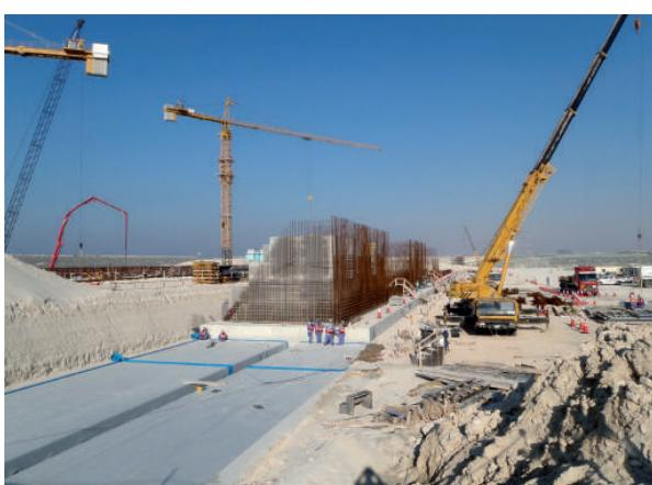
Emirates Nuclear Energy Corporation (ENEC) is developing the first nuclear power plant in the UAE. The project site area is **80** hectares where it is planned to build 4 Power Plant Reactors. The specification required a 47,000m<sup>2</sup> waterproofing system for the substructure. Fosroc specified Proofex PGP which was approved and successfully applied.
